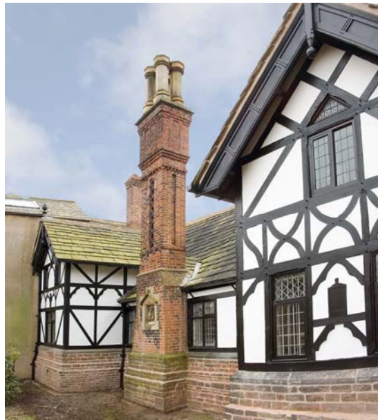
Part of the Restored Timber Work from the 2004/05 Project
